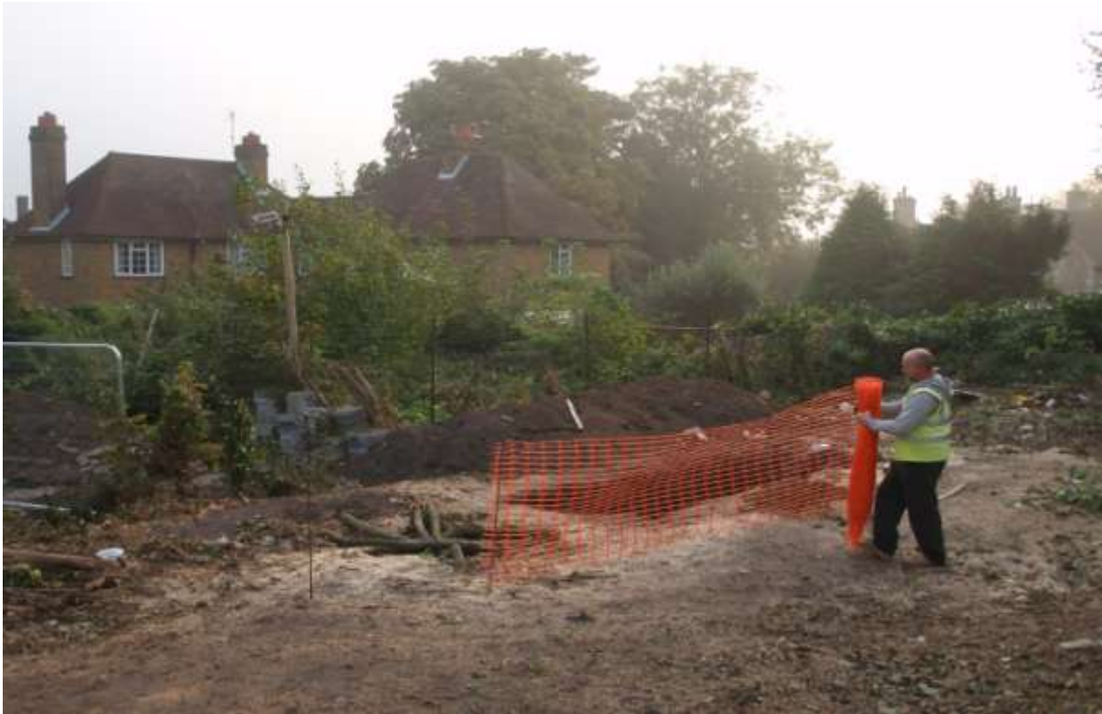
Plate 2 – Location shot of trench, looking north-east.
