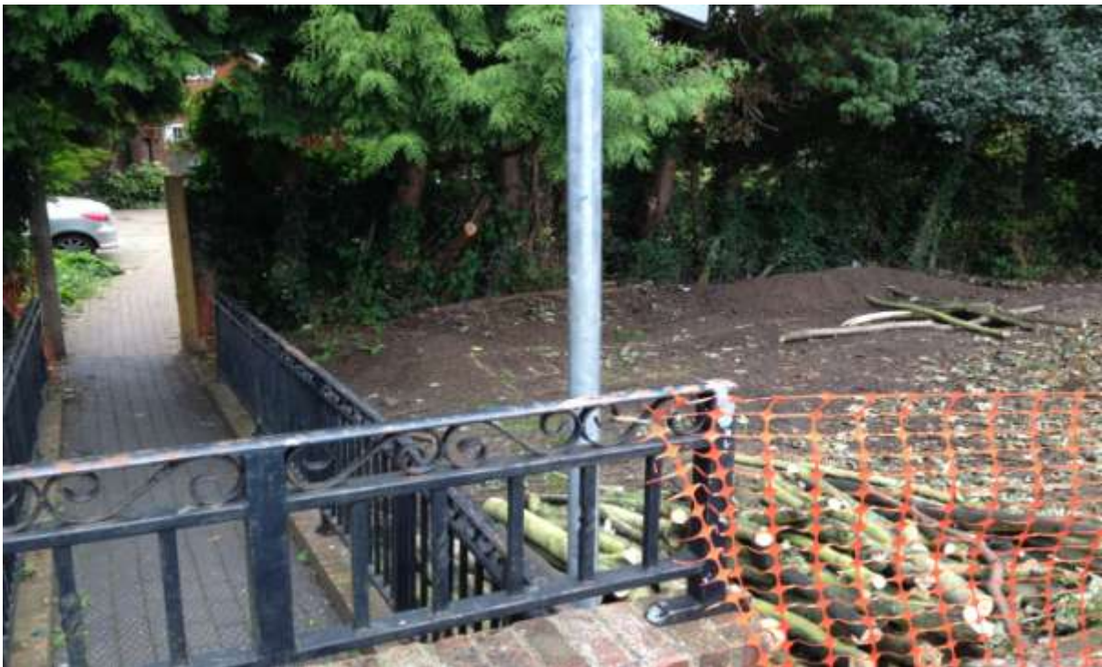
Plate 3 – View of site looking at area of Trench 3
